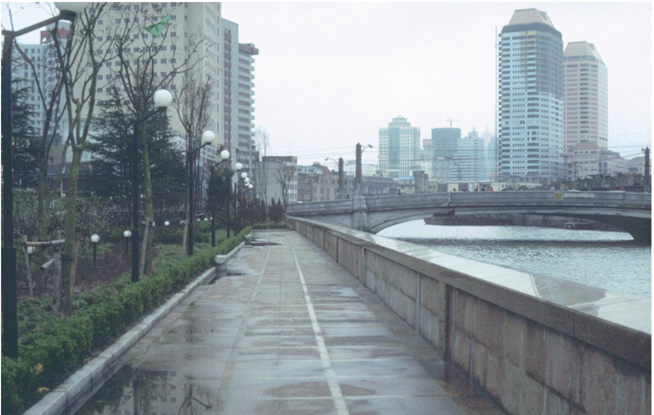
Renewal of Suzhou Creek embankment and flood wall. (photo: Peter Kerssens)
