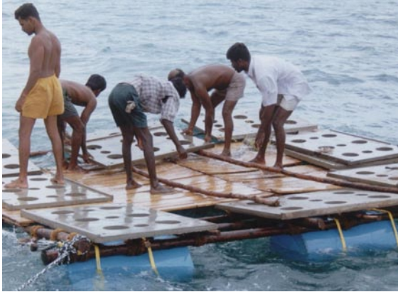
Figure 1: Module design, transport of modules parts (slabs) on rafts & assembling the modules parts to the deployment in three locations at a water depth between 3.2 and 5.6 m. (photos: SDMRI)
