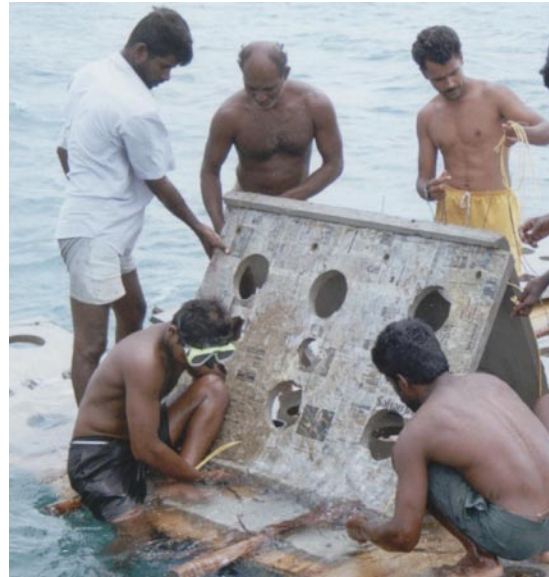
Figure 1: Module design, transport of modules parts (slabs) on rafts & assembling the modules parts to the deployment in three locations at a water depth between 3.2 and 5.6 m. (photos: SDMRI)
