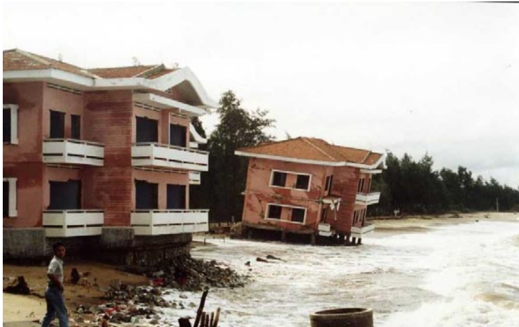
Figure 7: Coastal erosion Thuan An, TTHue Province, due to the November 1999 typhoon. (photo: R.Misdorp)
