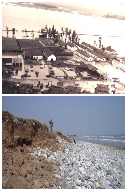
Figure 6: Nam Dinh Province: salt panning behind the sea-dike in a polder; ongoing coastal erosion and flooding; eroded and flooded & ruined village with remnants of church towers; sea-dike toe erosion. (photos: Hans Pos, VNICZM project)
