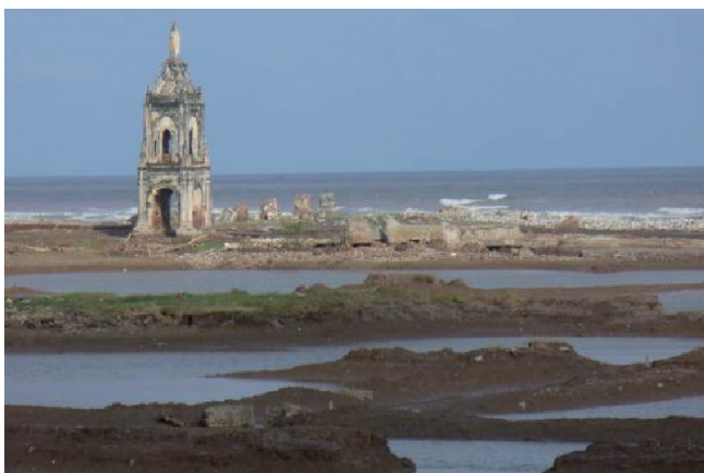
Coastal dynamics play an important role along the Vietnamese coastline. Here in Nam Dinh, part of the Red River Delta coast, complete villages have disappeared due to coastal erosion. (photo: G.J. Schiereck)
