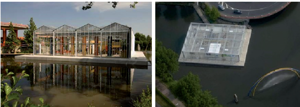
First - built floating greenhouse in the world - Demonstration version, municipality of Westland (photos: Dura Vermeer).
