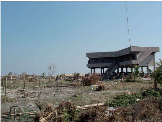
A cyclone shelter in Dublar Char, Bangladesh, recently withstood a cyclone and saved many lives. (photo: Gerhard Tauscher, International Federation of Red Cross & Red Crescent)
