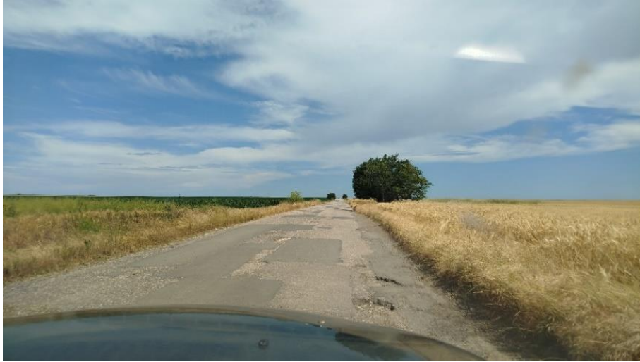
Figure 6. - The stage of the road which connects Vadu to Corbu
